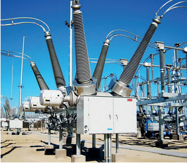
SF 6 Gas Circuit Breakers Dead Tonk Type BAKS
